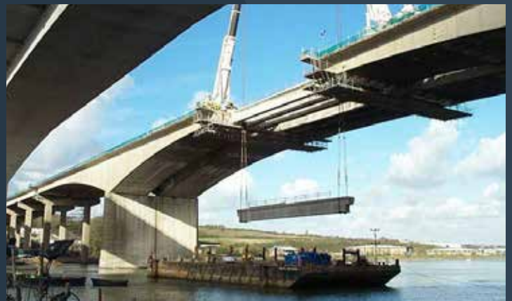
Existing Medway Bridge, UK
