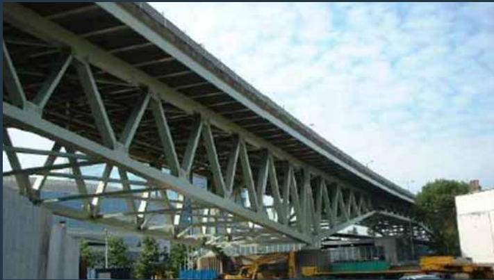
Boston Manor Viaduct, UK
