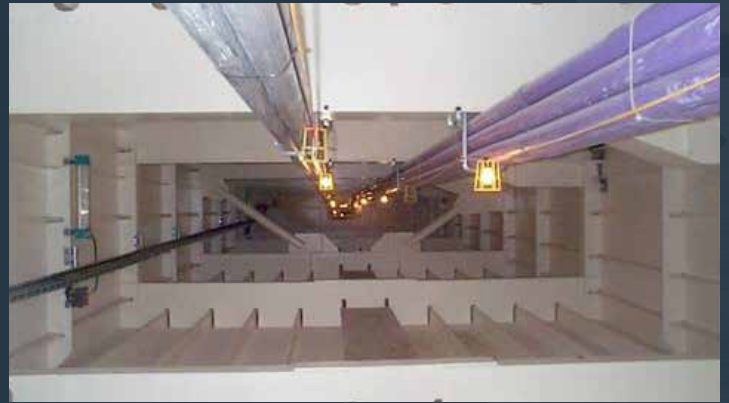
Avonmouth Bridge, UK
